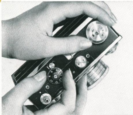
After advancing the film as explained in Step 5, set Counter Dial by turning it counter-clockwise (to the left) until "O" is opposite index line. The Counter Dial indicates the number of pictures taken. The camera is now ready for the first picture.
