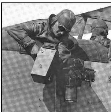
From 1919 Photographic Review . Camera held on its side, next to fixed mounted camera.
