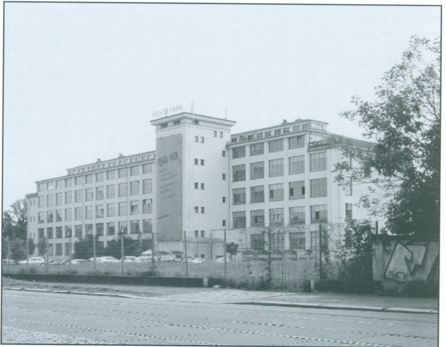
The ICA-Werke , also in Dresden. This building is where ICA cameras were made before the "Zeiss Ikon" merger, and Contax cameras afterwards. It has been turned into an office building called "Pentapark."
