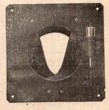
side, and the shutter requires no setting, as it works automatically, setting itself after each exposure without opening the wings, and is always ready.
