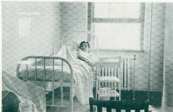
Single Hospital Room Through Wire Glass.
