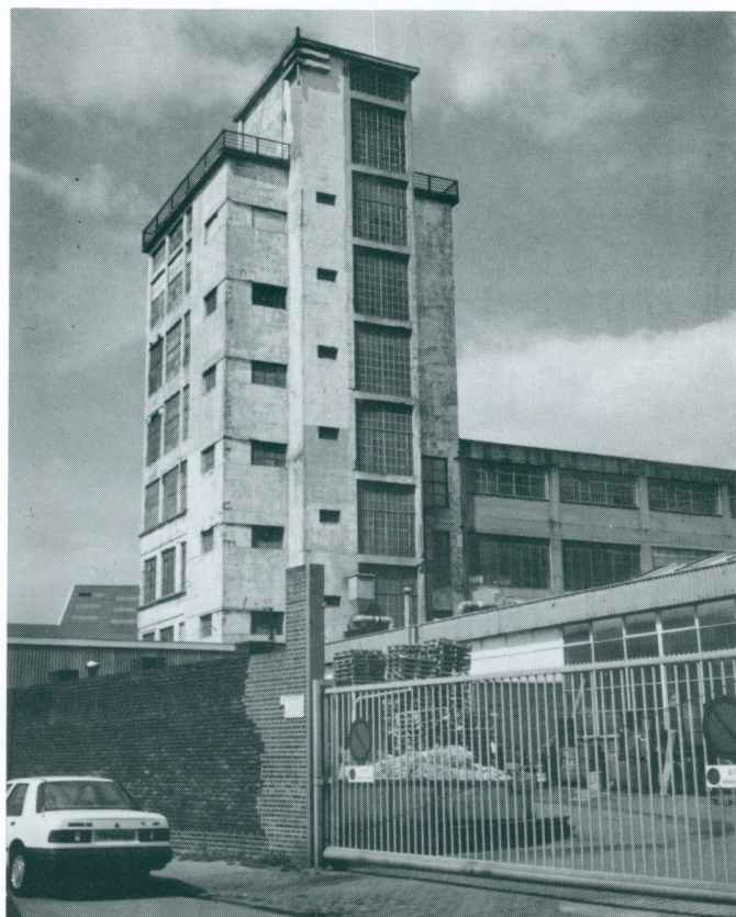
The Nedinsco plant's tallest structure: used to test long optical instruments such as periscopes prior to shipment.
