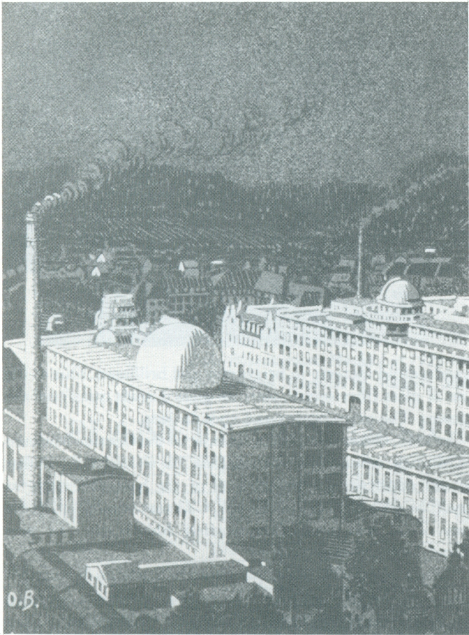
Carl Zeiss Jena, 1926 view of the factory. At far left is the dome for testing the first planetarium projector. The other dome tested telescopes.
